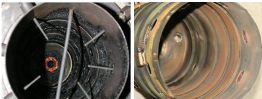
Figure 2: Flame tube interior. Left: Original flame tube. The sediments on the walls are clearly visible. Right: Optimized flame tube. Note the clean flame tube without any sediment.
