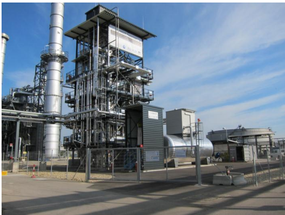
Figure 1: The integrated pilot plant at OMV refinery Schwechat.
