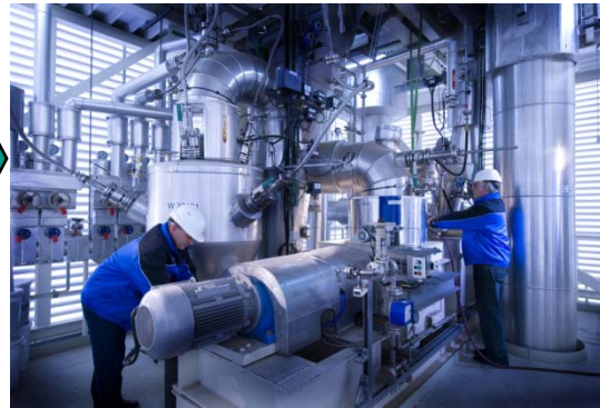
Fast pyrolysis reactor
