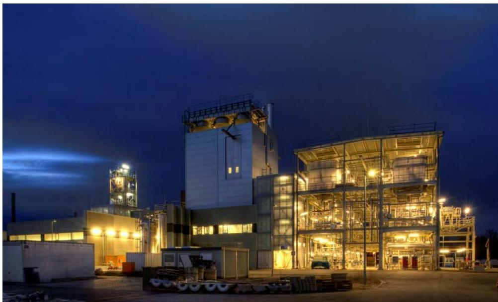
**Figure 1:** The bioliq pilot plant at the KIT in Karlsruhe, Germany, has a straw pyrolysis unit of 500 kg/h (2 MW) with bioslurry preparation, an high pressure, entrained flow gasifier with a capacity of 1 t/h bioslurry (5 MW) with hot gas cleaning and fuel synthesis unit operating at 55 bar.
