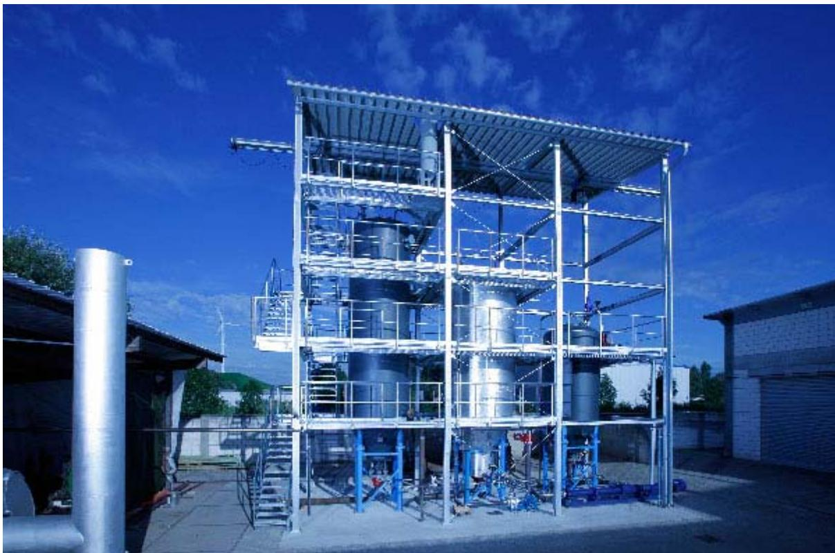
Figure 2: The world-wide first HTC-plant with commercial-scale reactors at AVA-CO2 with a nameplate capacity of 8400 t/a biomass residues from breweries, municipalities and agriculture.
